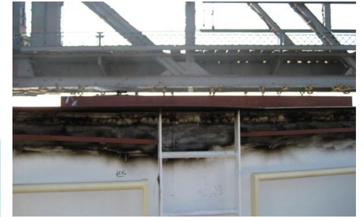
Clearance between cut funnel and bridge
