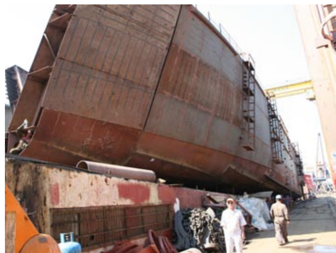
Manager Mr. Gokmen with Hull No. 33 under construction
